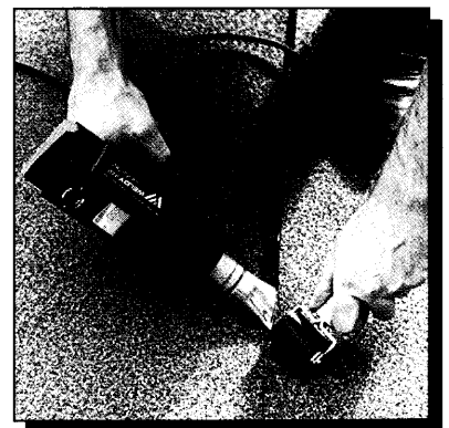
Welding bitumen and roofing felt
